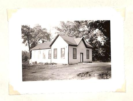
A one story, detached, frame building with metal roof, on stone foundation, containing two rooms, heated by stoves, the flues to which are of standard construction, lighted by electricity. This building is approximately 26' X 72' and is in poor condition, the walls appear to have buckled and the floor has dropped down slightly.
