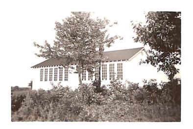
A one story, frame building with metal roof, on concrete foundation. This building contains only one room, is heated by a stove, the flue to which is of standard construction, is lighted by electricity. It is approximately  $31\frac{1}{2}$ ' X  $47\frac{1}{2}$ ' and is in excellent condition. This building is located approximately 43 feet west of the Aldie new shoool.
